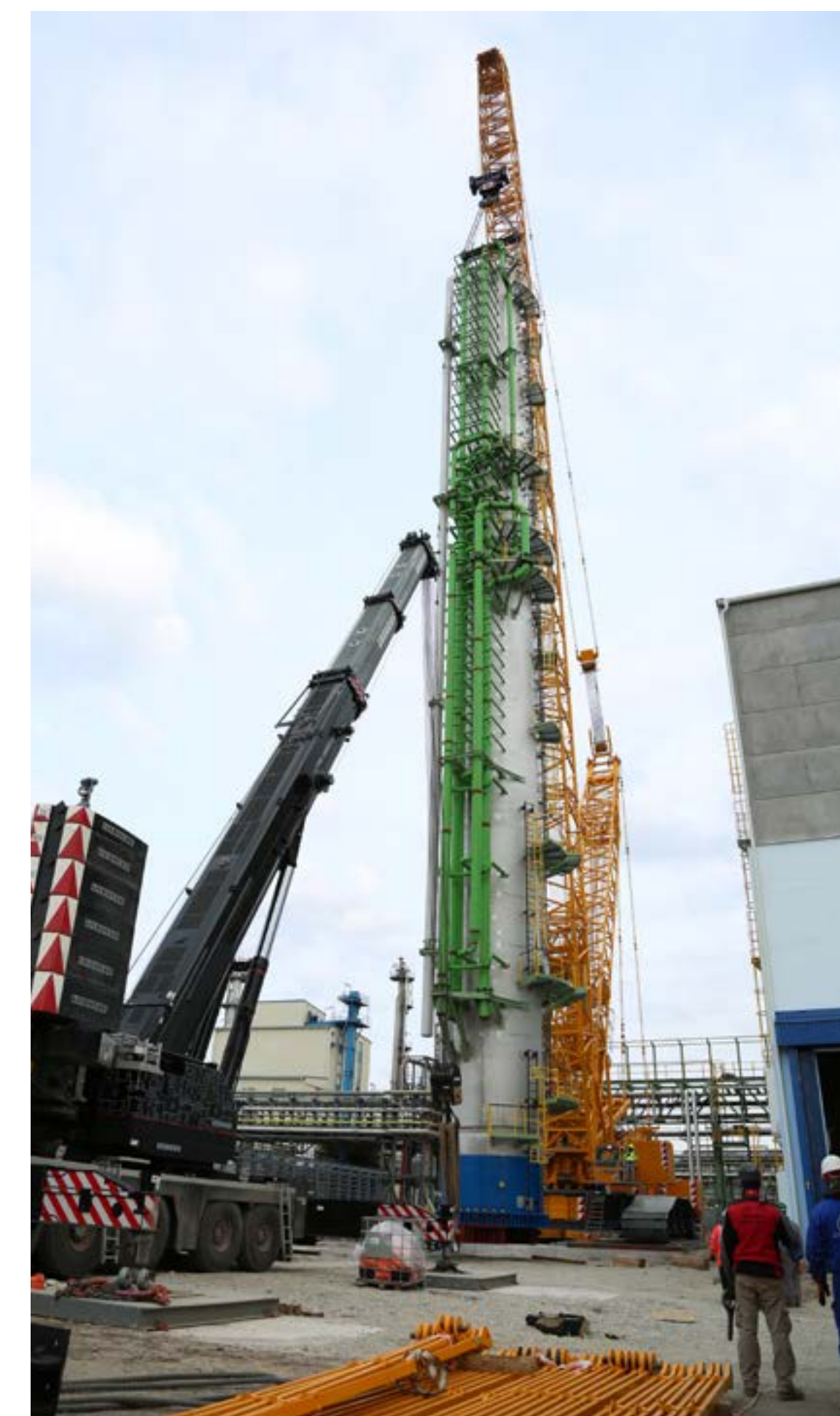
Installation of the absorption column
