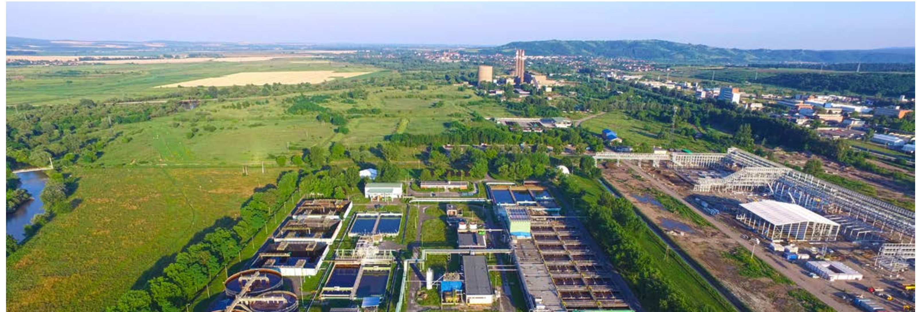
Wastewater Treatment Plant, BorsodChem
