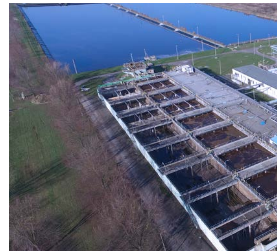
Wastewater Treatment Plant, BorsodChem
