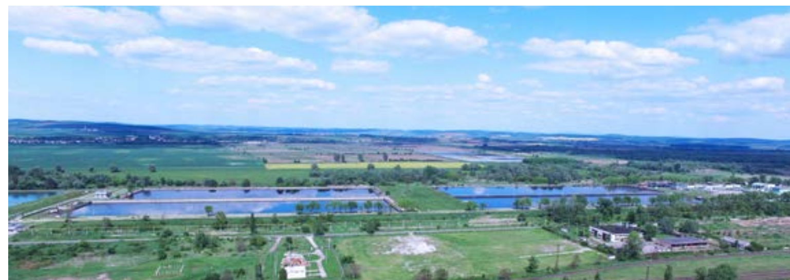
Wastewater Treatment Plant, BorsodChem
